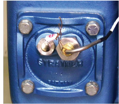
Figure 5-3. Dual Port Strainer Cover
