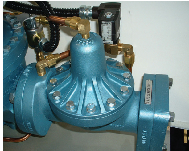
Figure 3-5. Dual Stage LPG Valve
